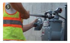
Hand tighten the outlet swivel cap. Using a pipe wrench, alternate between both swivel caps and tighten approximately three flats (approximately 20 ft/lb). DO NOT OVER TIGHTEN. Damage to the rubber gasket inside the swivel cap may result. 6 Check all connections for leaks.
