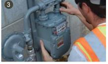
Inlet and outlet pipe connections should be parallel. The height difference between the housing connections should be no more than 1/4".
