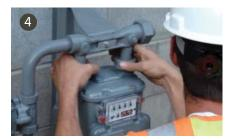
Hand tighten the inlet swivel cap. Pressurize the system to purge the air inside the meter through the outlet. Please note that the line from the meter to the appliance(s) must also be purged prior to lighting.
