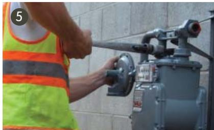
Hand tighten the outlet swivel cap. Using a pipe wrench, alternate between both swivel caps and tighten approximately three flats (approximately 20 ft/lb). DO NOT OVER TIGHTEN. Damage to the rubber gasket inside the swivel cap may result.
