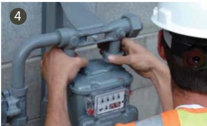
Hand tighten the inlet swivel cap. Pressurize the system to purge the air inside the meter through the outlet. Please note that the line from the meter to the appliance(s) must also be purged prior to lighting.
