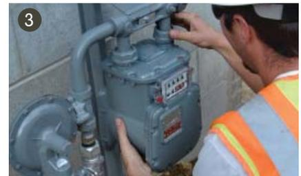
Inlet and outlet pipe connections should be parallel. The height difference between the housing connections should be no more than 1/4".
